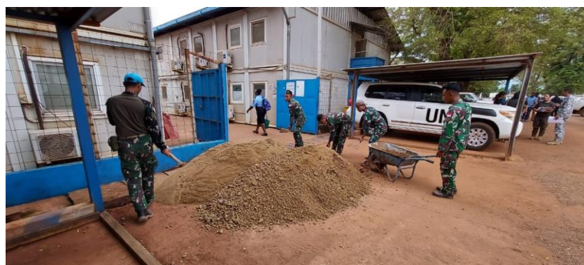
Figure 6. Construction of an FC garage at UCATEX
