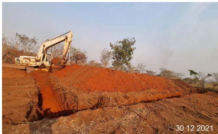
Figure 4. Trench and Embankment Work at Carnot
