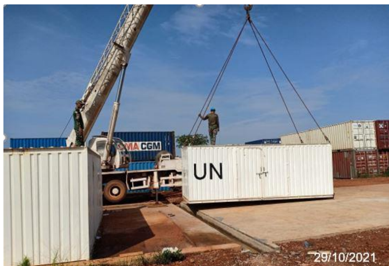
Figure 1. Crane Work for Shifting Incinerator at CWH M'Poko
